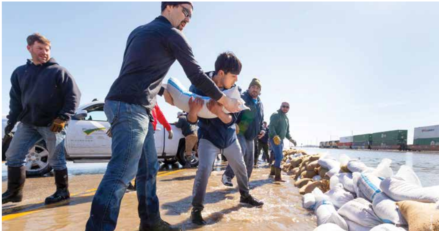
Volunteers race to stave off floodwaters by sandbagging along Old U.S. Highway 275 in Dodge County, Neb. Photo by Kent Sievers/The World-Herald; used with permission
