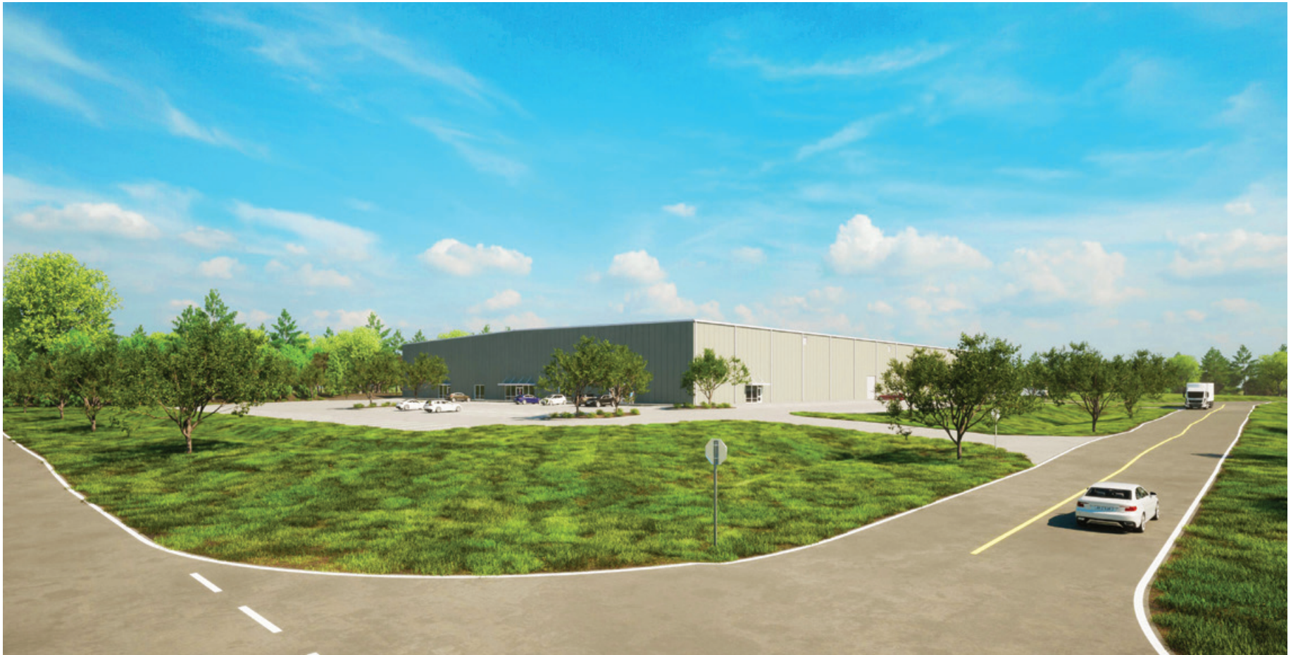
Nash County, N.C. is attracting new businesses to its county with shell buildings and completed surrounding infrastructure. An artist's conception shows one such building.
