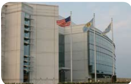
New Castle County, DE Public Safety Building
