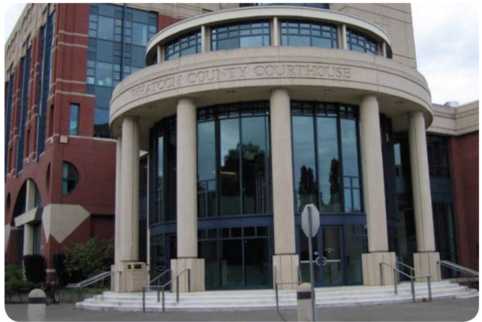
Whatcom County, WA Courthouse
